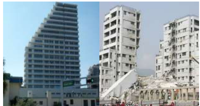
Figure 1: Irregular building the collapse of irregular buildings due to the earthquake in Islamabad
